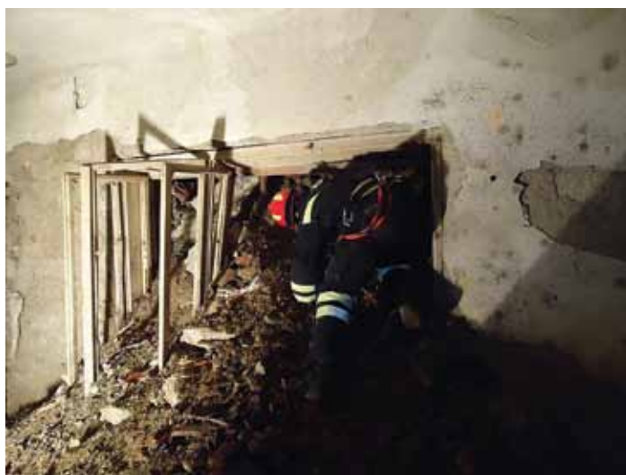
Figure 2. Collapse site search (Photo: Z. Gorički)
