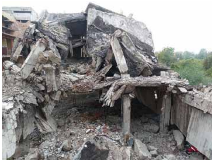
Figure 1. Collapse as a result of the combat activities in the war zone (Photo: Z. Gorički)
